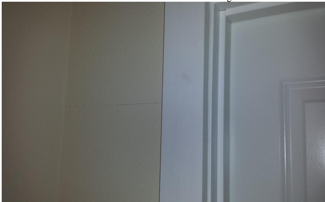
Structural / Shear-wall related damage
