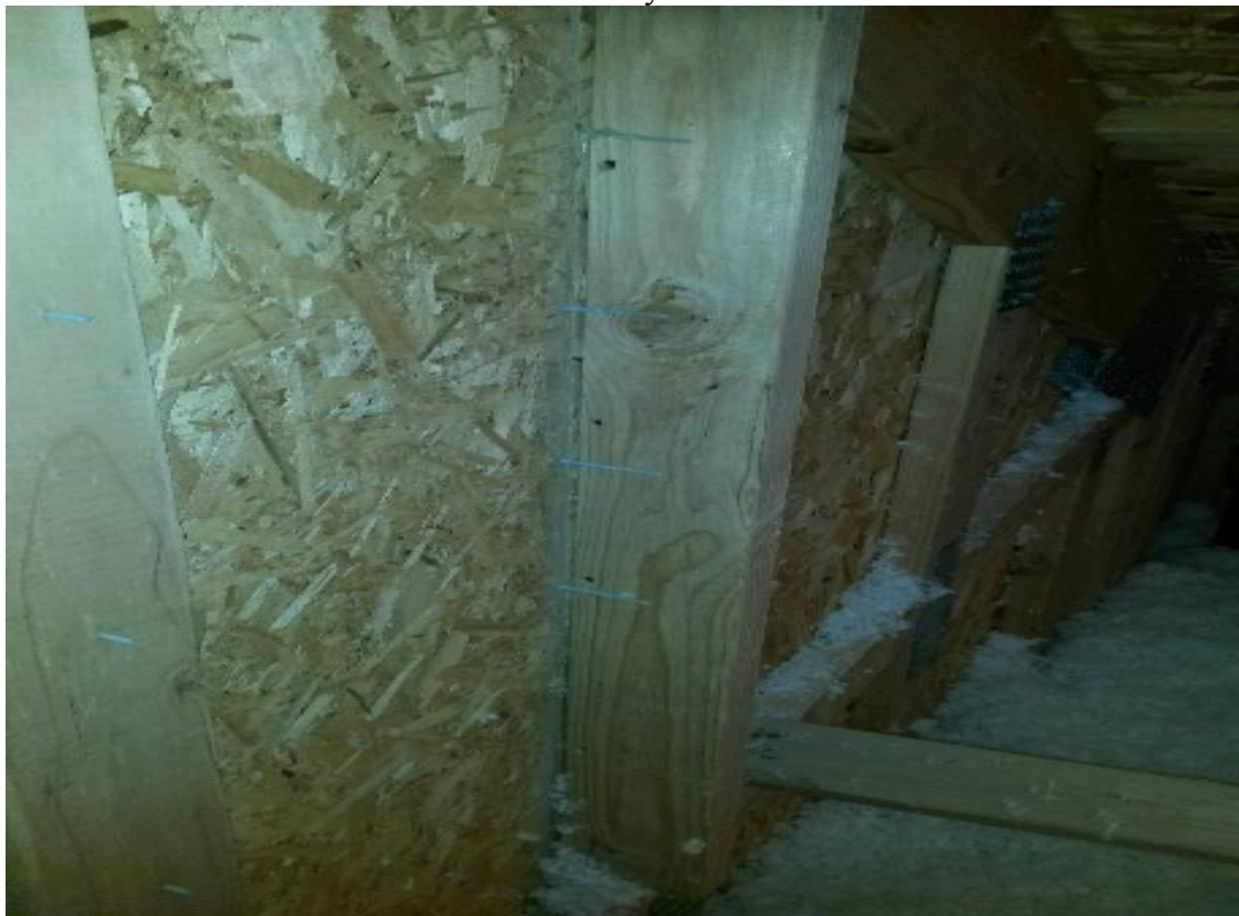
T-111 shear-walls incorrectly sized and left unsecured
