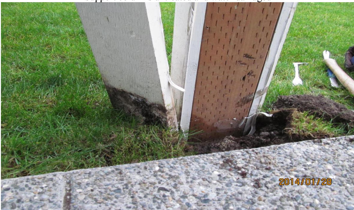
Support columns untreated and water damaged
